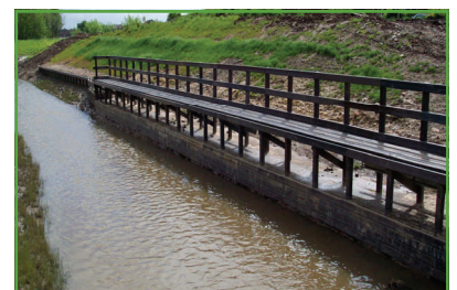
i-plas profiles used to create a landing station
