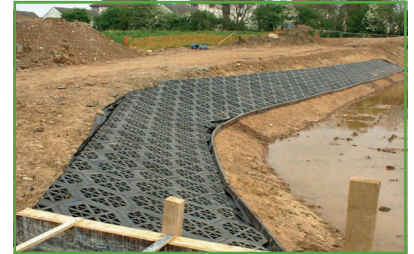
i-plas Groundblocks used as revetments
